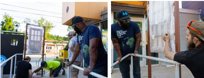
Installation of We Are Windows.
