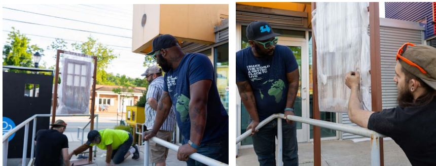
Installation of We Are Windows.
